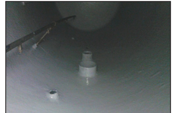
Coated tank internals
